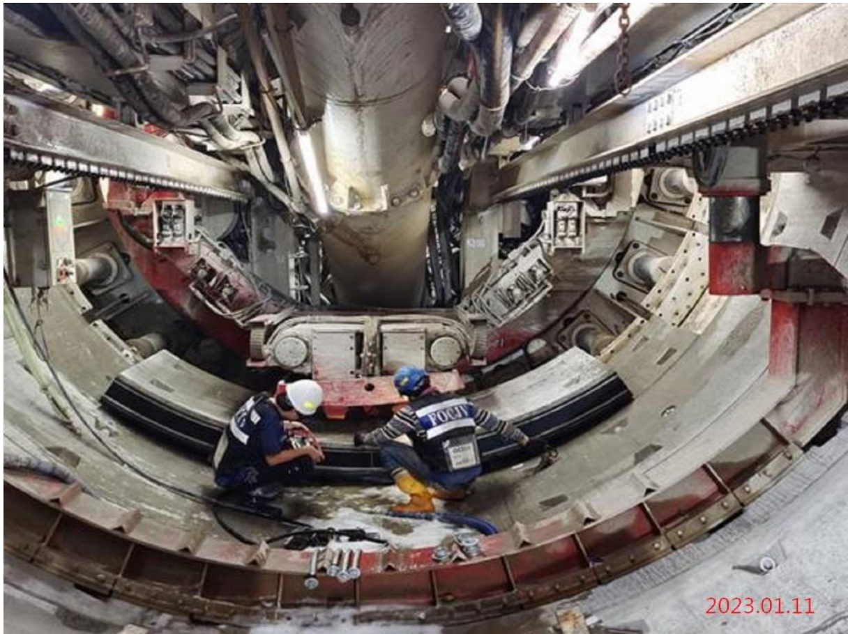
潛盾隧道_北出土段至 G12 站間小圓潛盾隧道掘進
