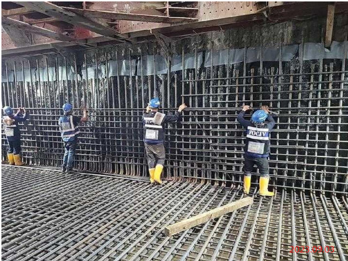
G10_南工區底版鋼筋綁紮
