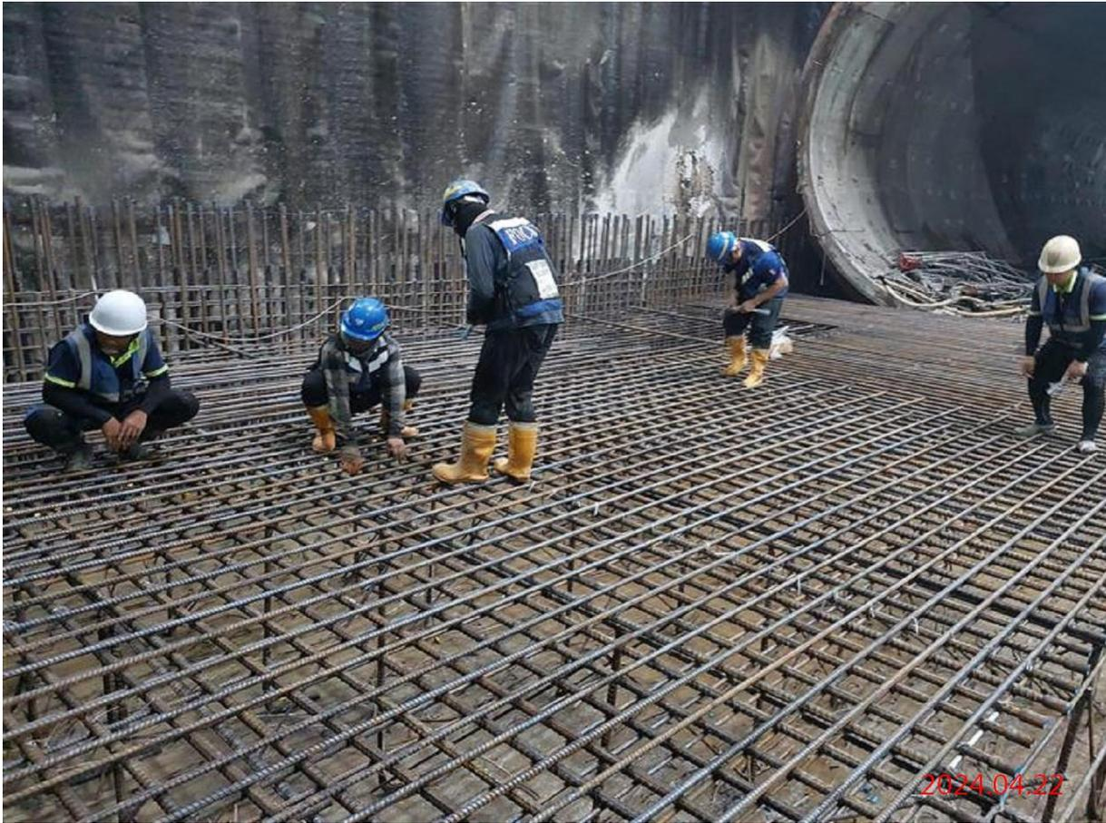
G11\_站體軌道層底版(下行線)鋼筋綁紮
