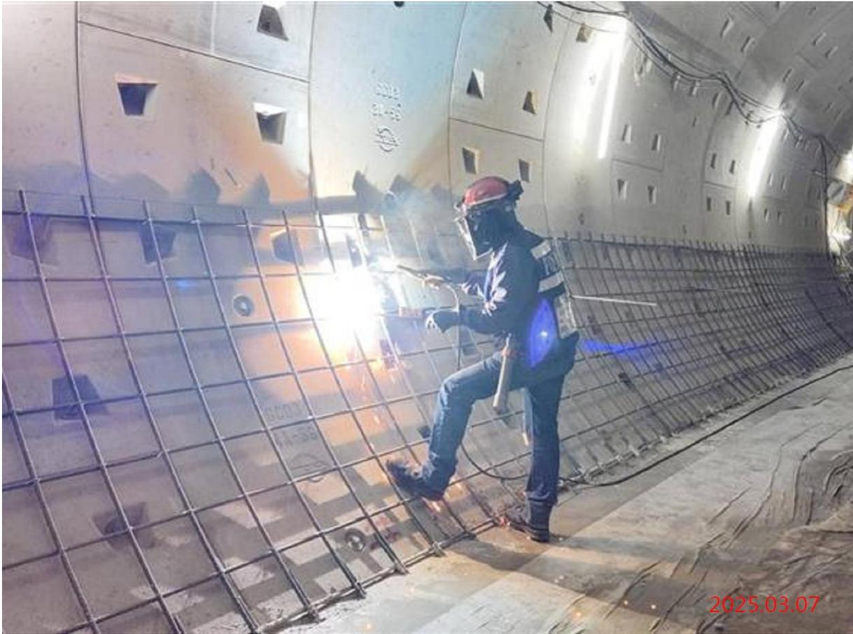
潛盾隧道\_G11~G12 下行線步道樣架電焊作業
