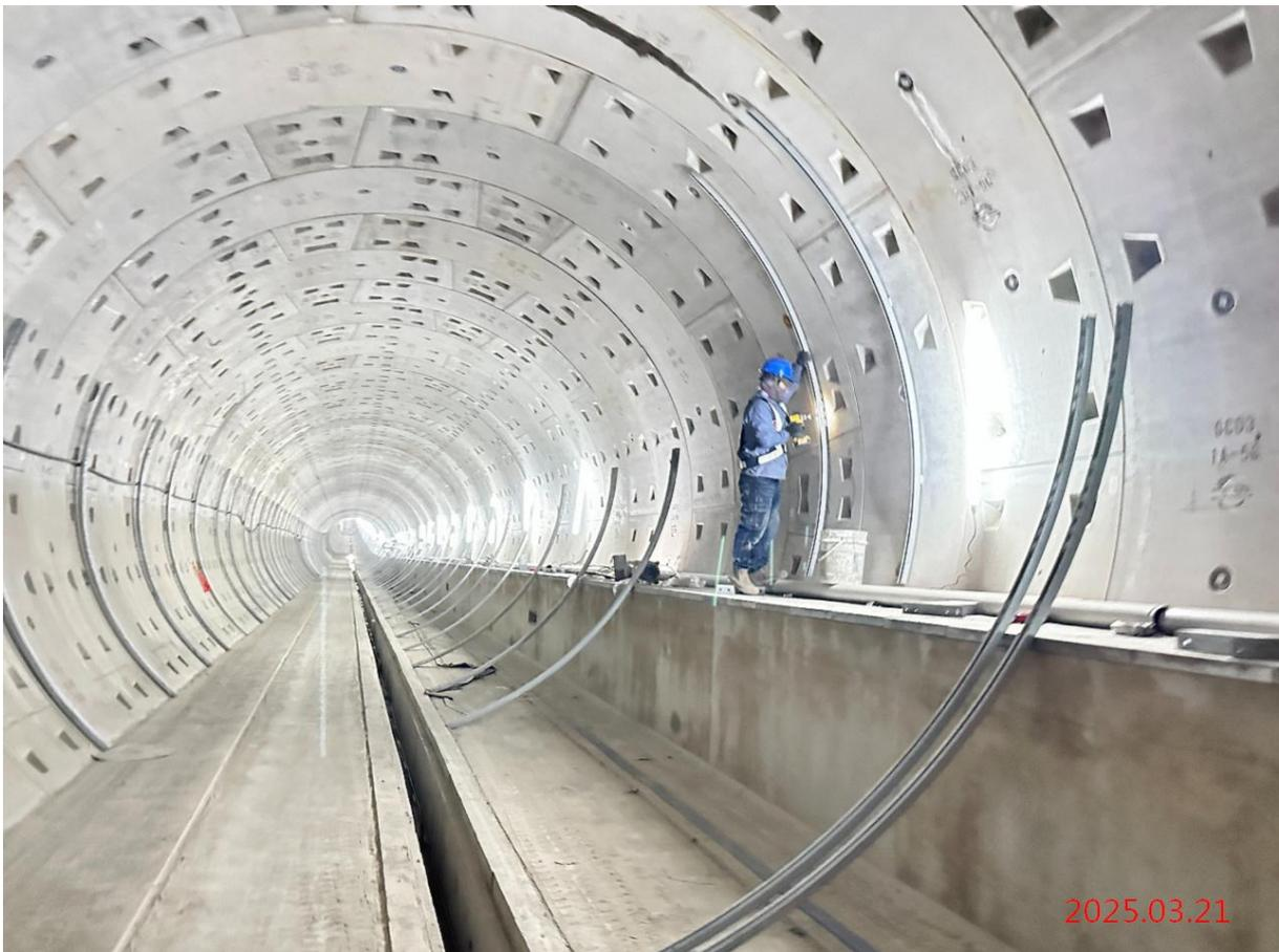
潛盾隧道\_G12~北出土段下行線滾邊槽鋼安裝
