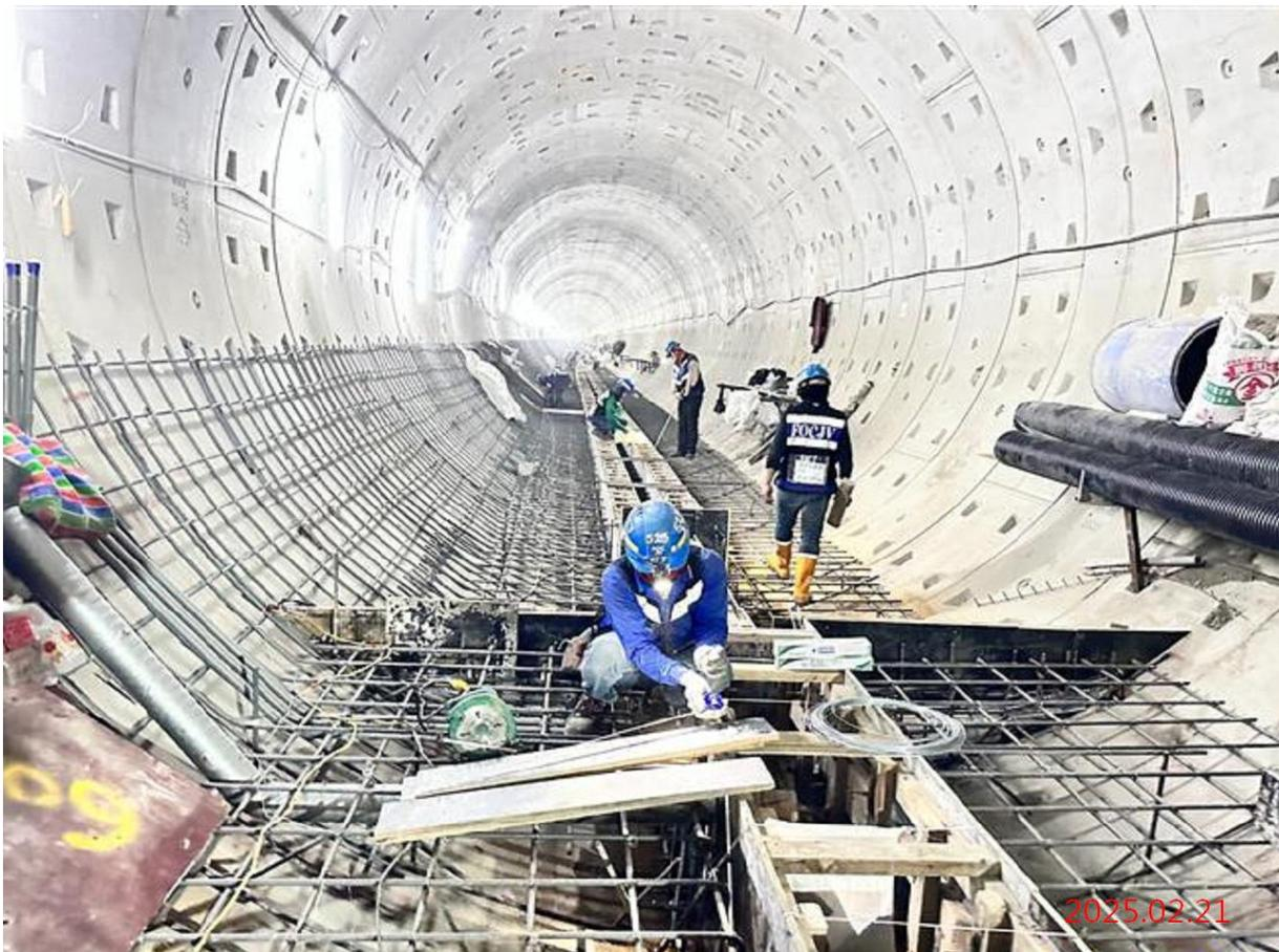
潛盾隧道\_G11~G12 下行線仰拱水溝模板組立
