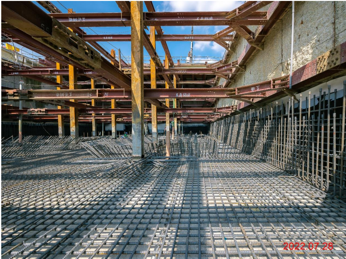
G12 站_站體穿堂版鋼筋綁紮
