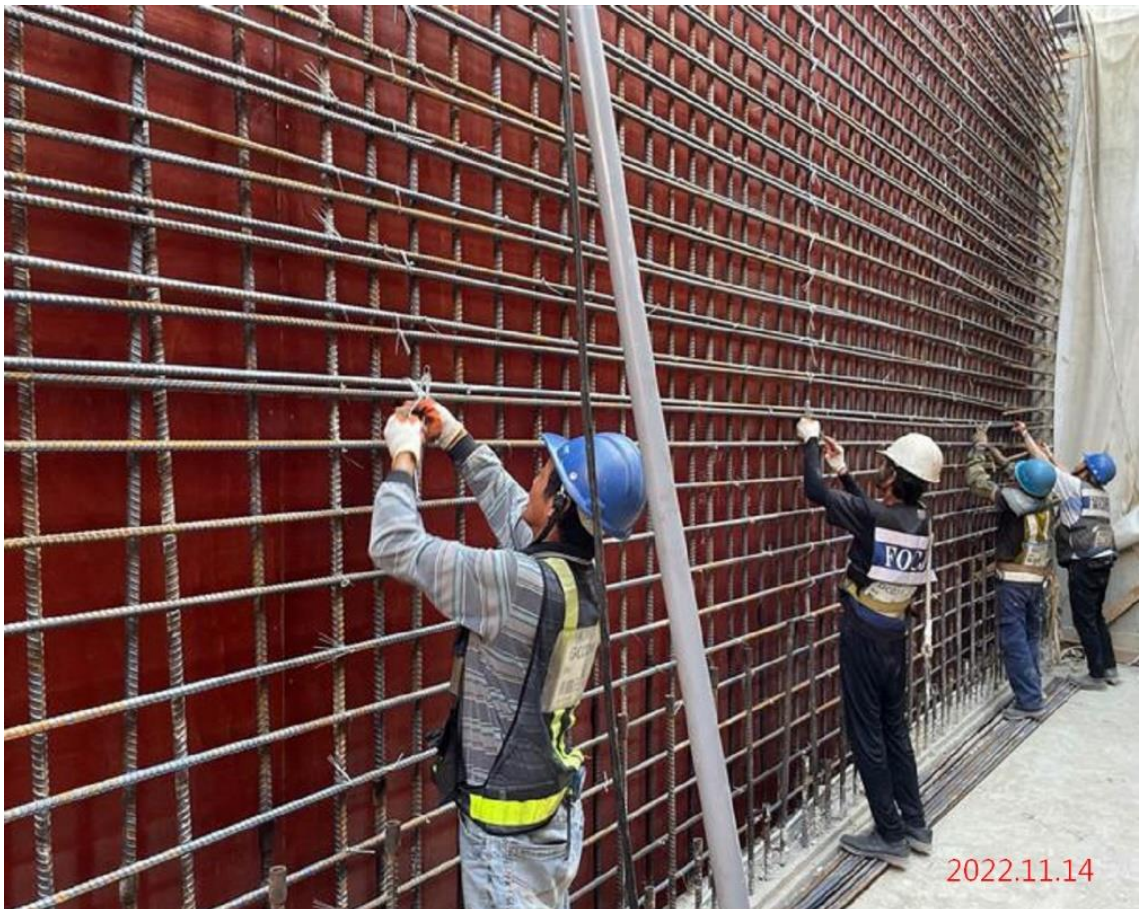
G12 站_承重牆鋼筋綁紮
