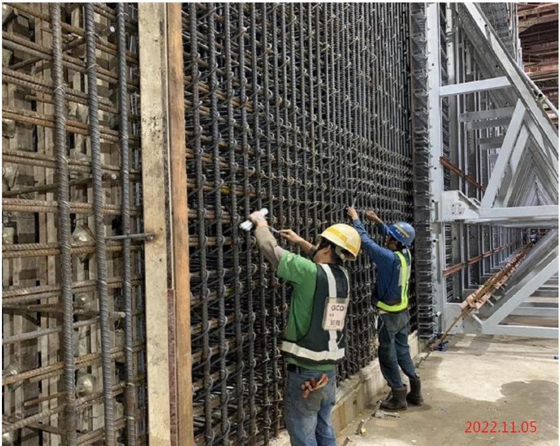
G11 站_站體側牆鋼筋綁紮
