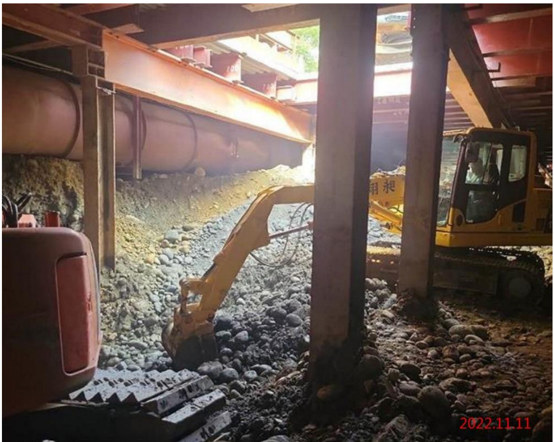
G10 站_站體開挖
