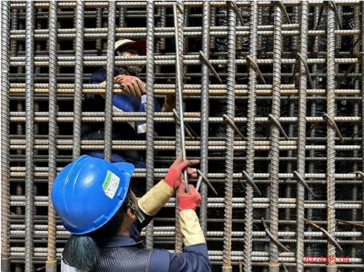
G10_站體穿堂層側牆鋼筋綁紮
