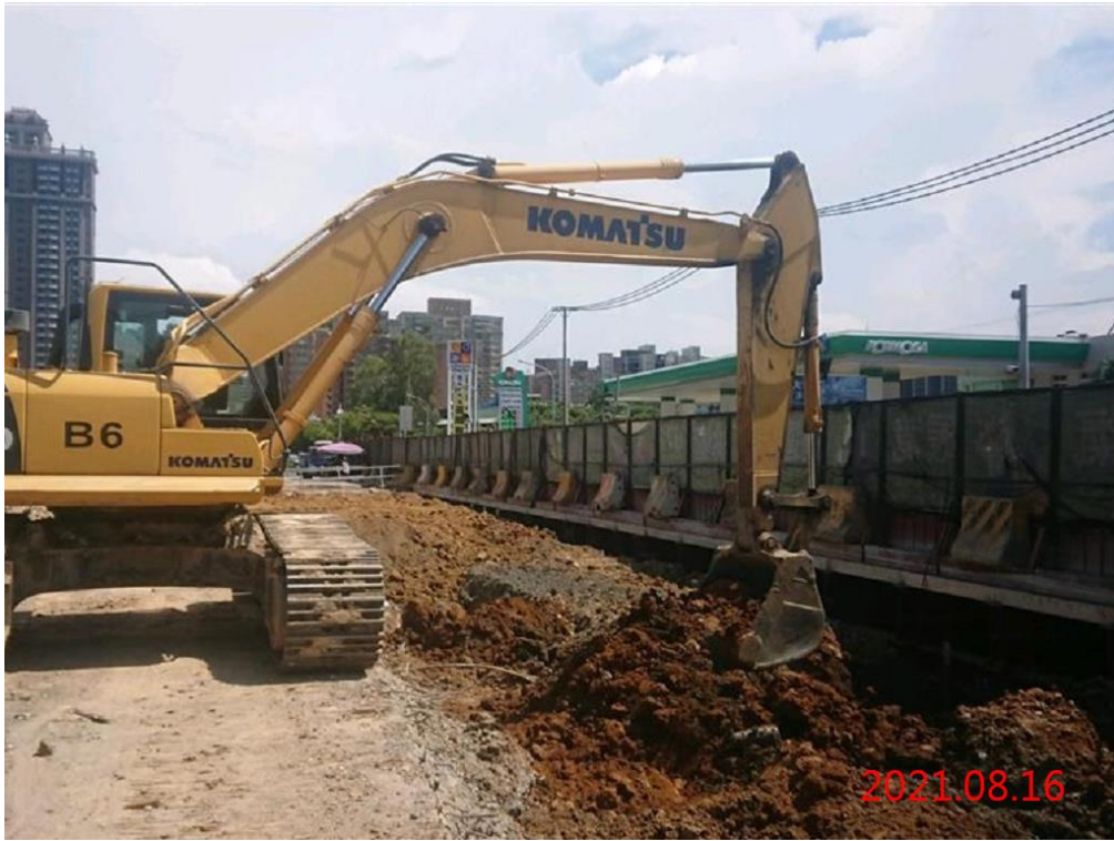
G12 站_站體開挖
