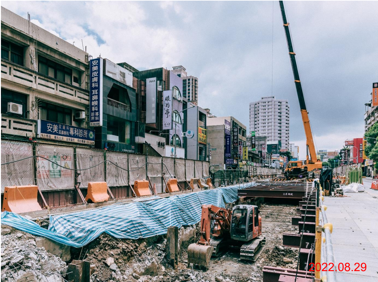
G10 站_站體開挖
