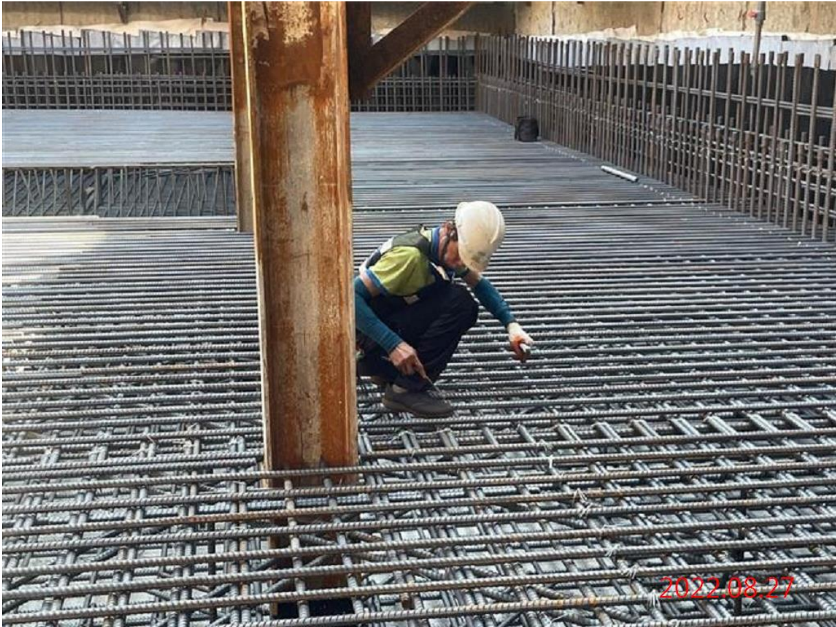
G12 站_站體底版鋼筋綁紮
