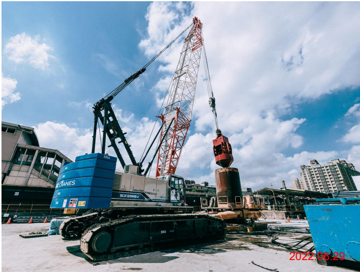
G07 站_全套管基樁抓掘
