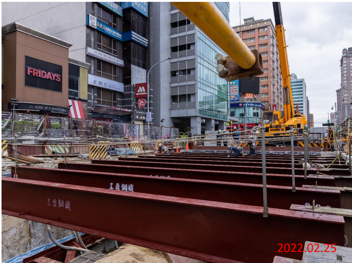
G11 站_站體淺挖及覆工
