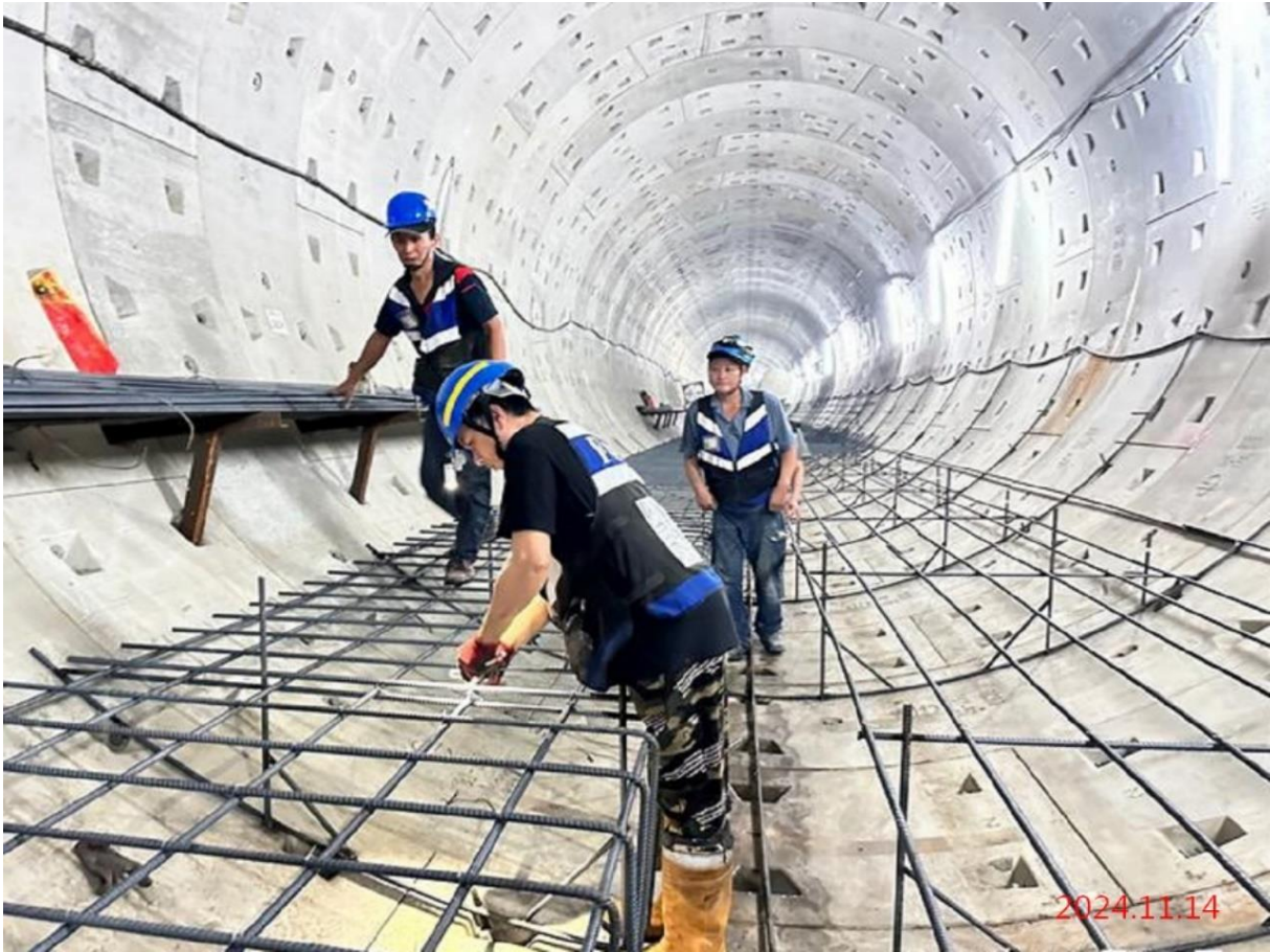
潛盾隧道_G12~北出土段下行線仰拱鋼筋綁紮
