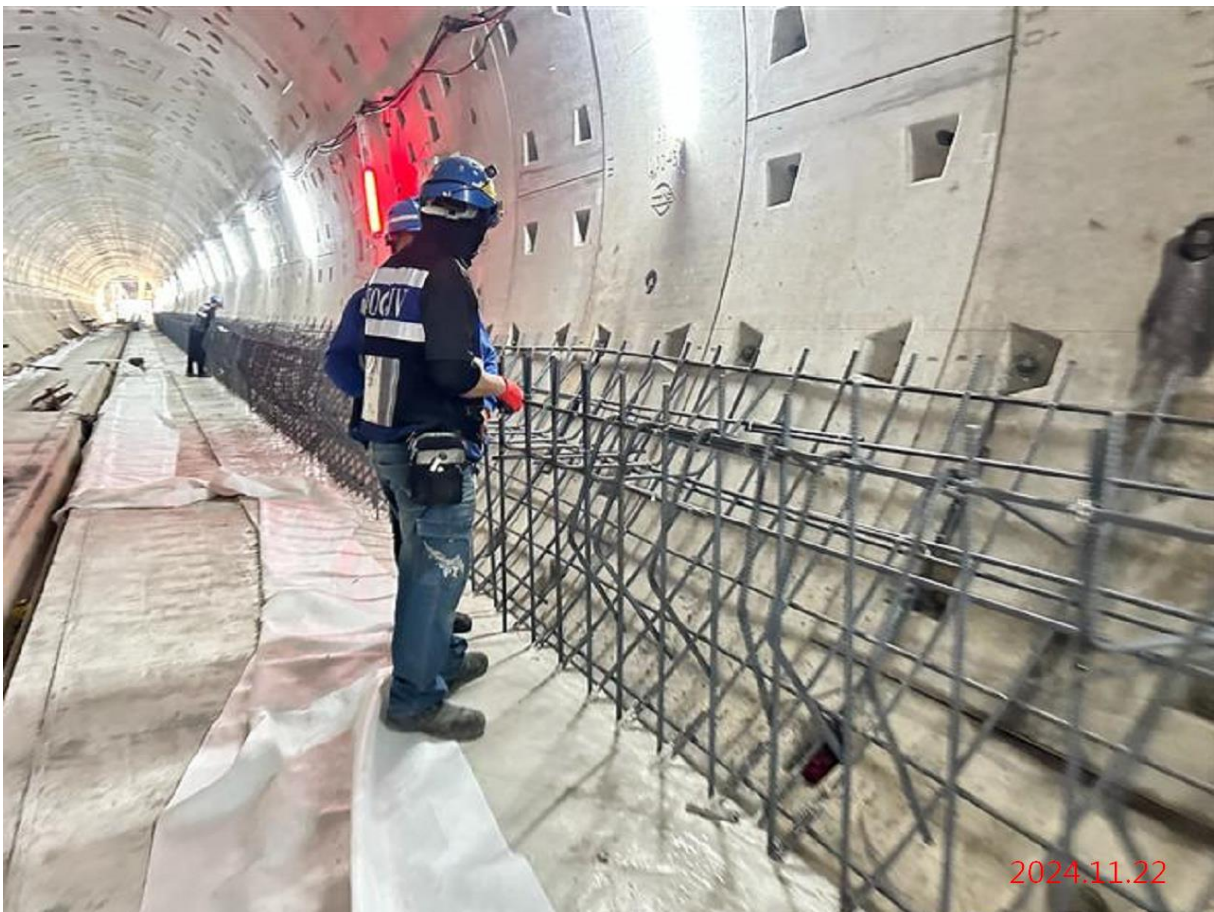
潛盾隧道_G12~北出土段下行線步道鋼筋綁紮
