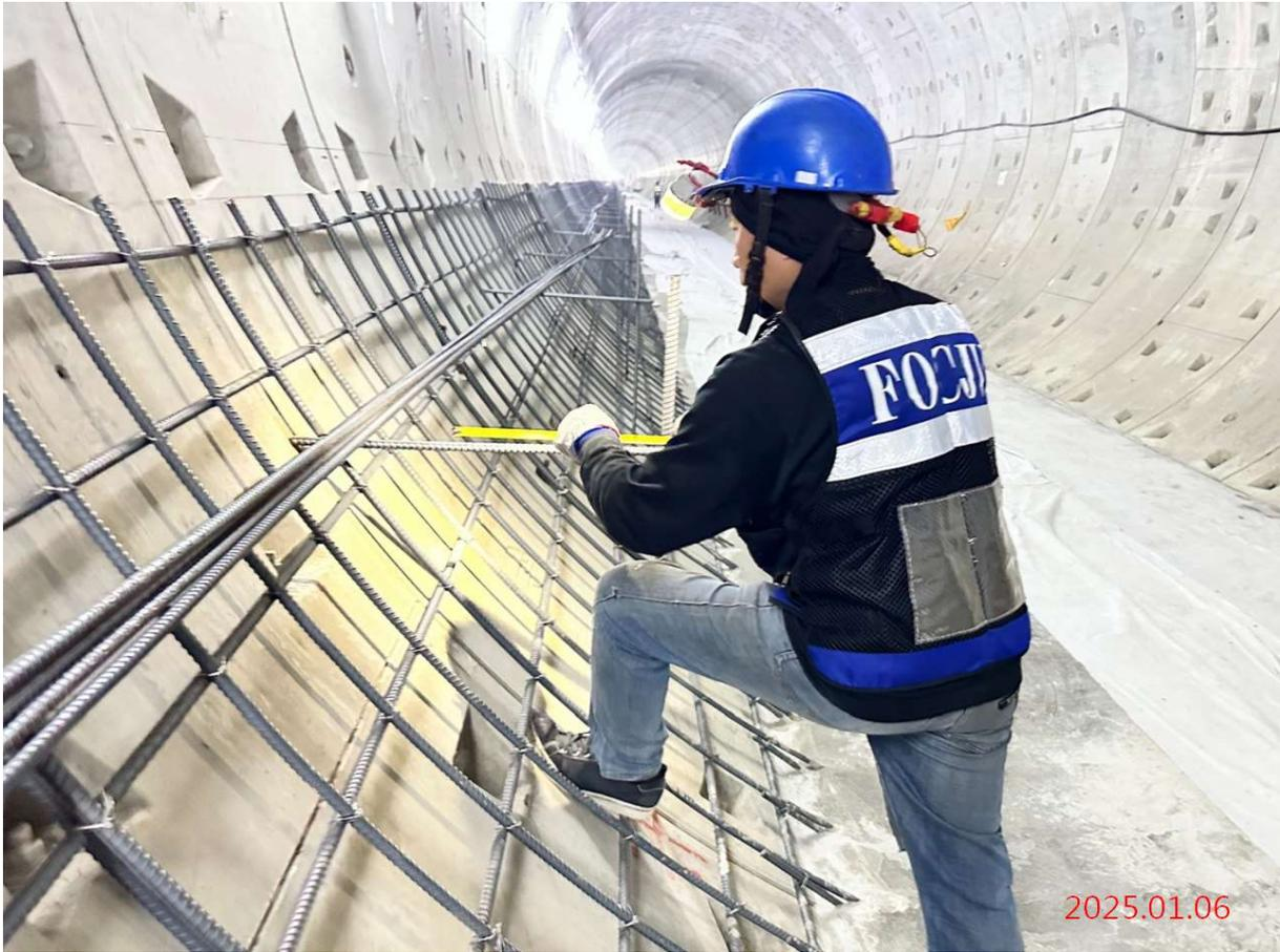
潛盾隧道\_G10~G11 下行線步道鋼筋綁紮
