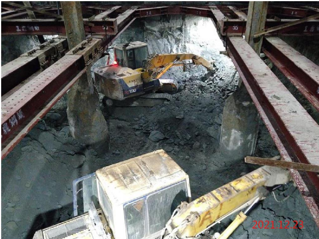
G12 站_站體開挖
