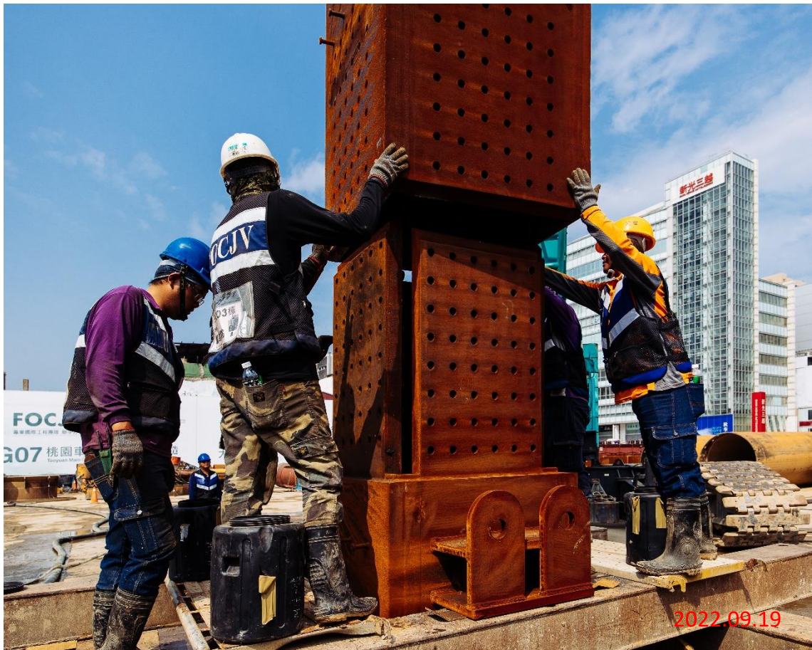
G07 站_全套管基樁逆打鋼柱搭接
