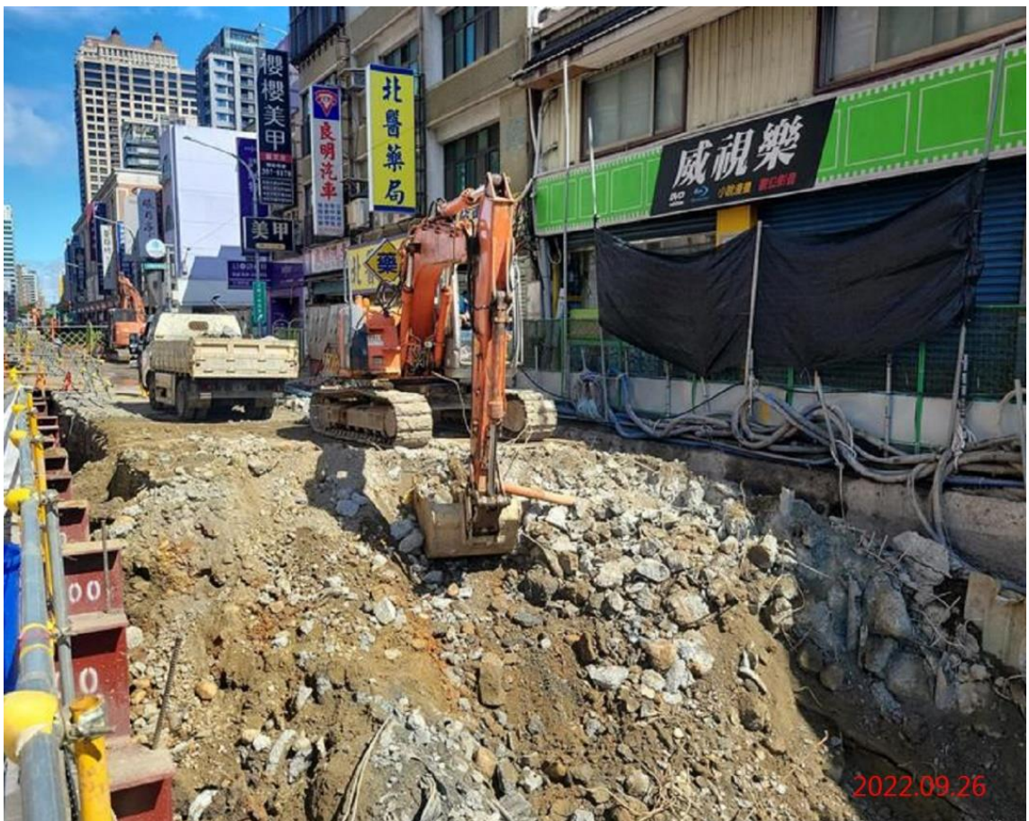
G10 站_站體開挖
