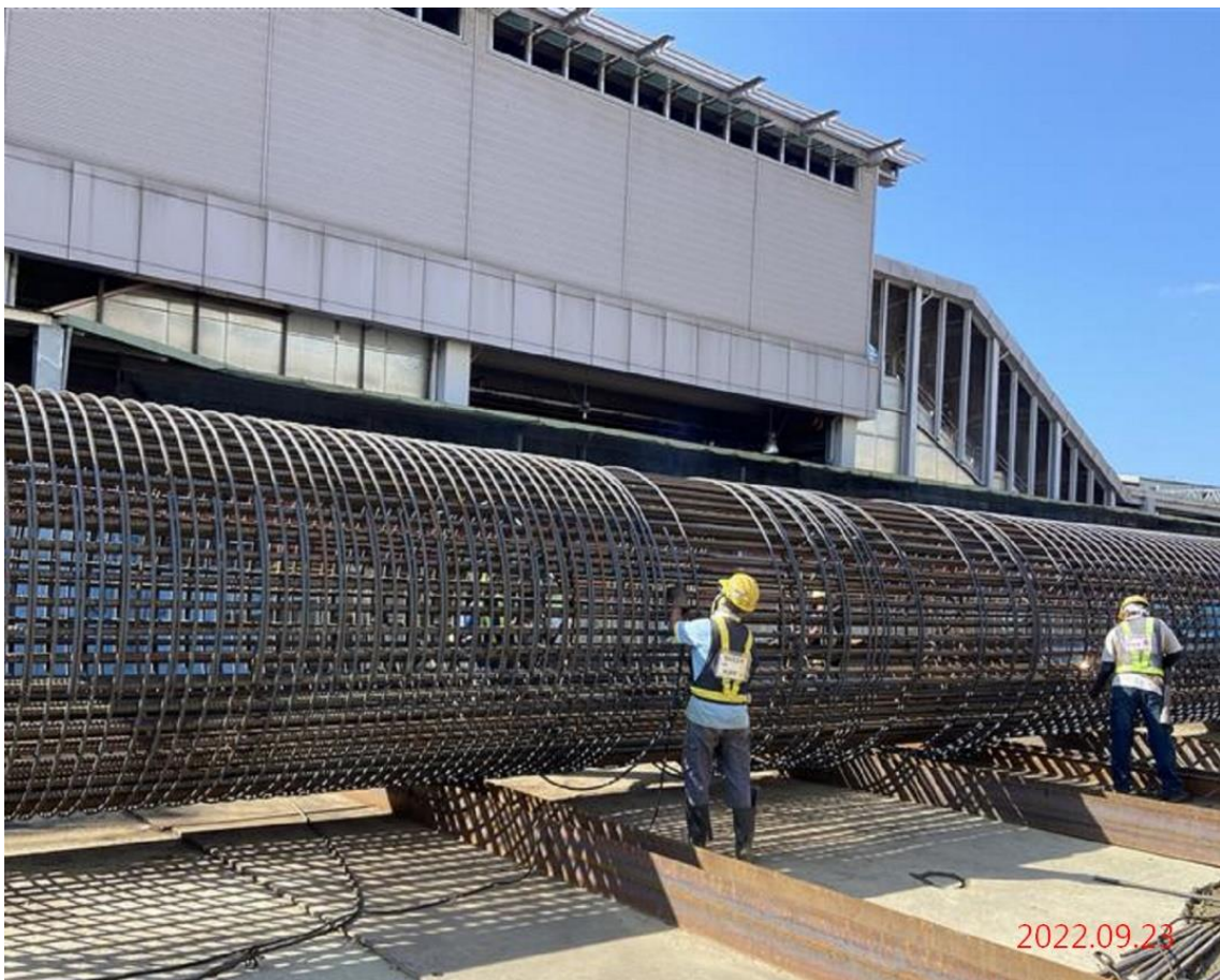
G07 站_全套管基樁鋼筋籠組立
