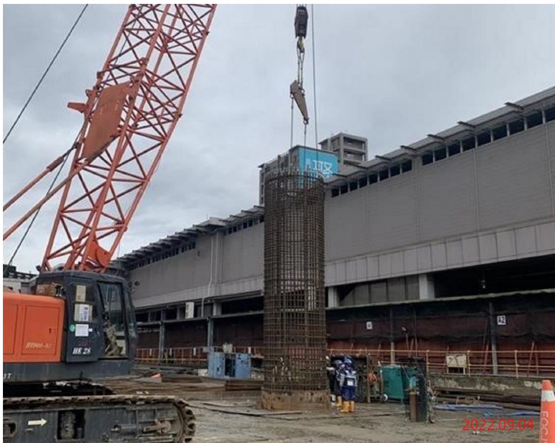
G07 站_全套管基樁鋼筋籠吊放
