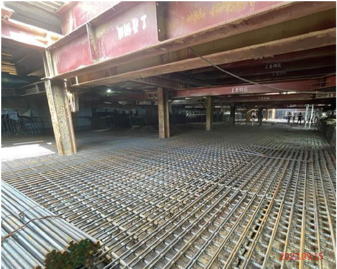
G12 站_站體頂版鋼筋綁紮
