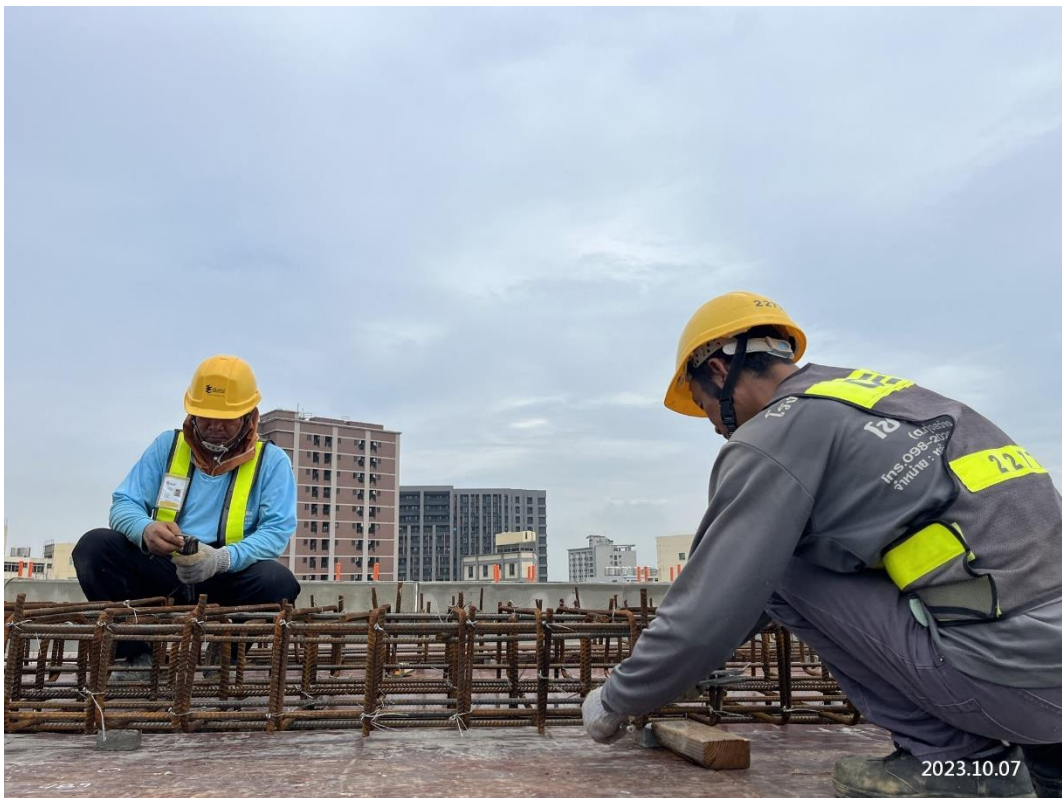
PDA-11~PD-10 中央步道鋼筋綁紮
