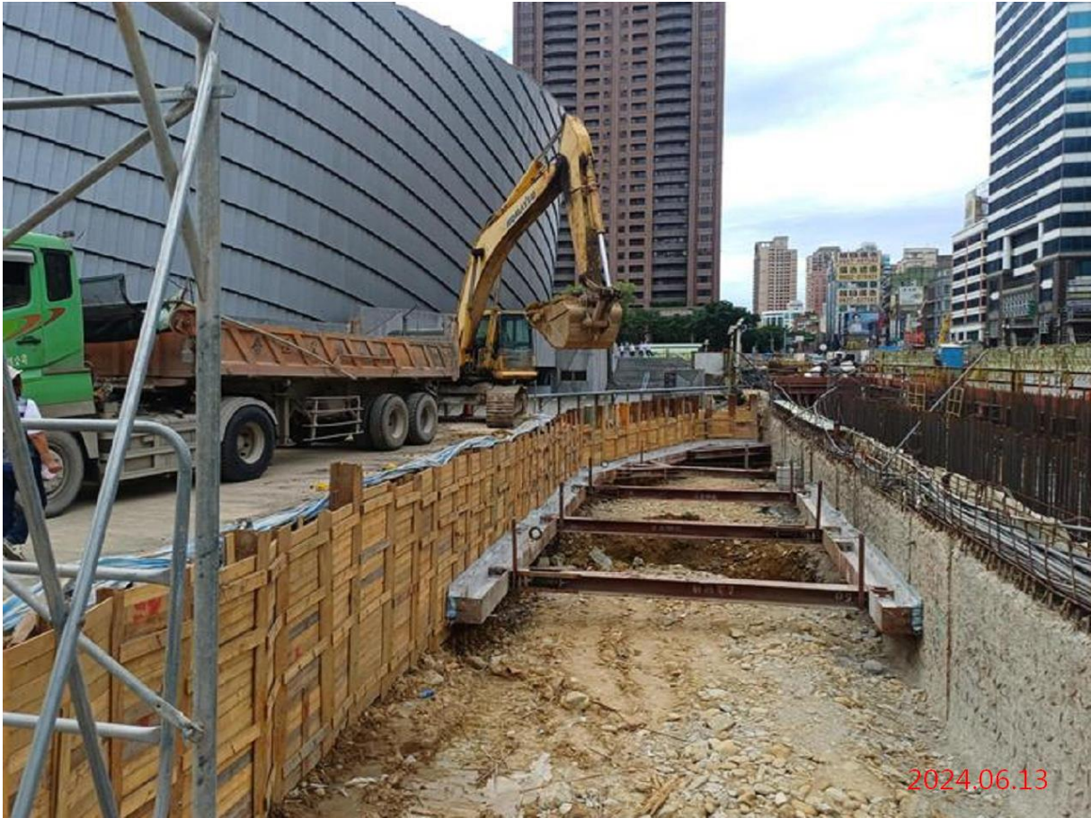
G11_出入口開挖
