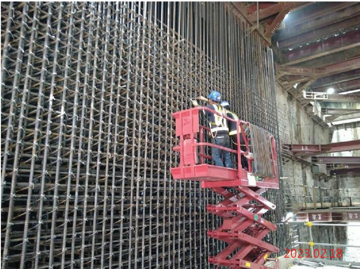
G11 站_站體穿堂側牆鋼筋綁紮
