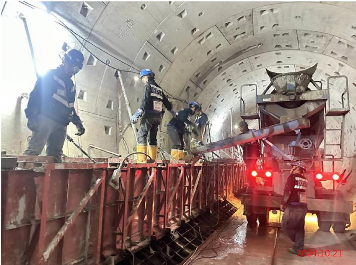
潛盾隧道\_G12~北出土上行線步道混凝土澆置
