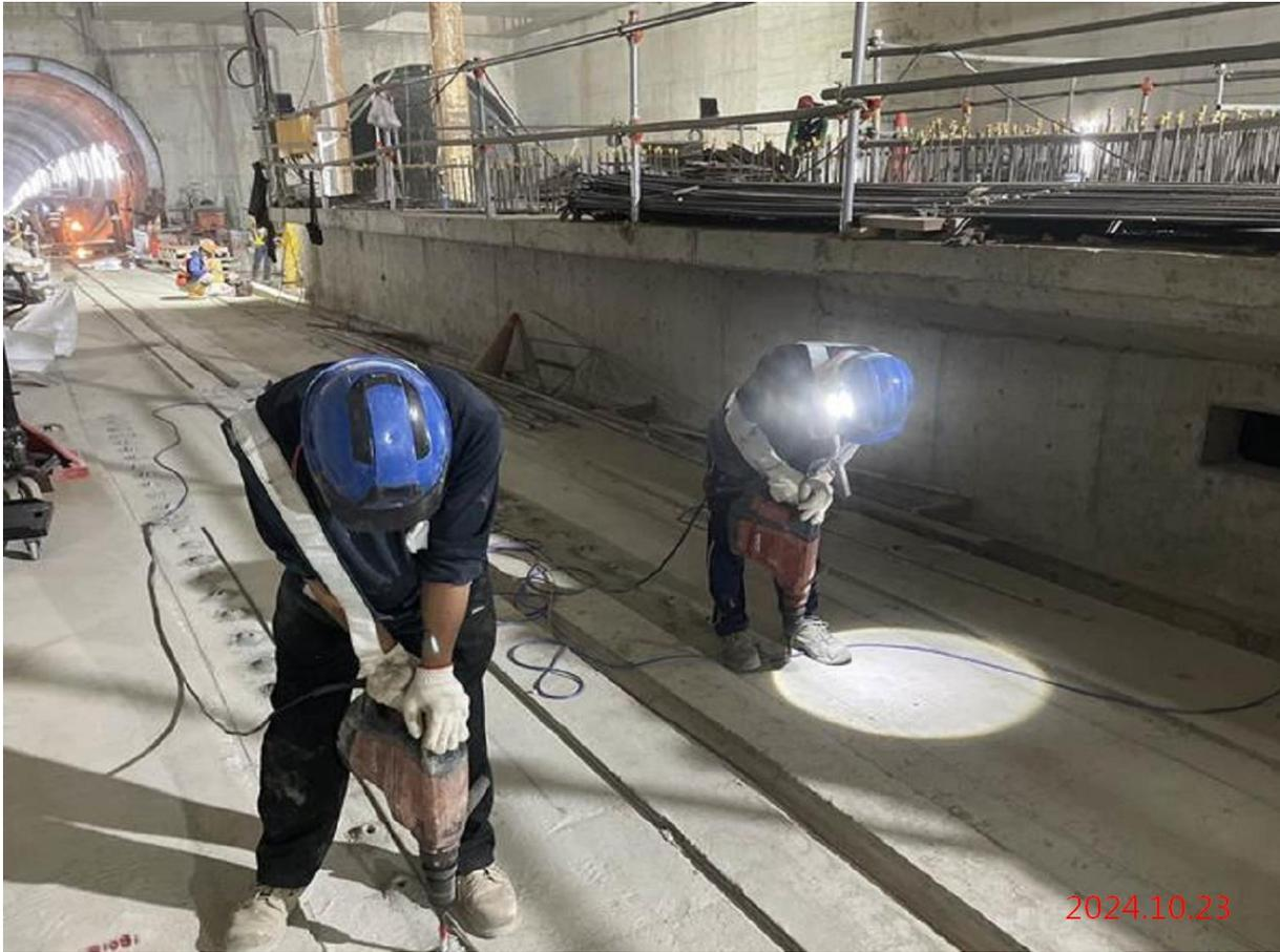
G12\_站體軌道層軌床道釘孔鑽孔
