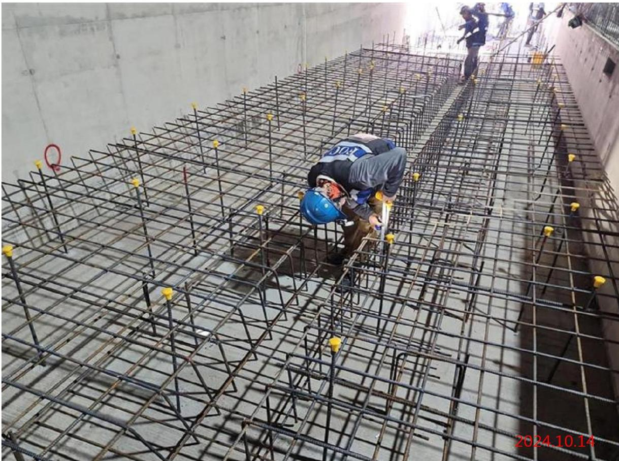
潛盾隧道\_G11~G10 仰拱樣架燒焊及鋼筋綁紮
