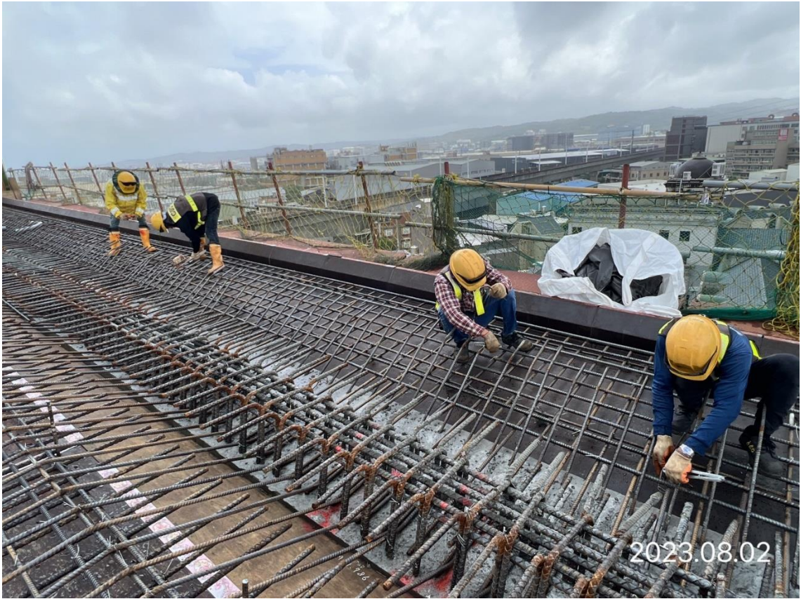
DU13a-10 場撐箱型梁頂版鋼筋綁紮
