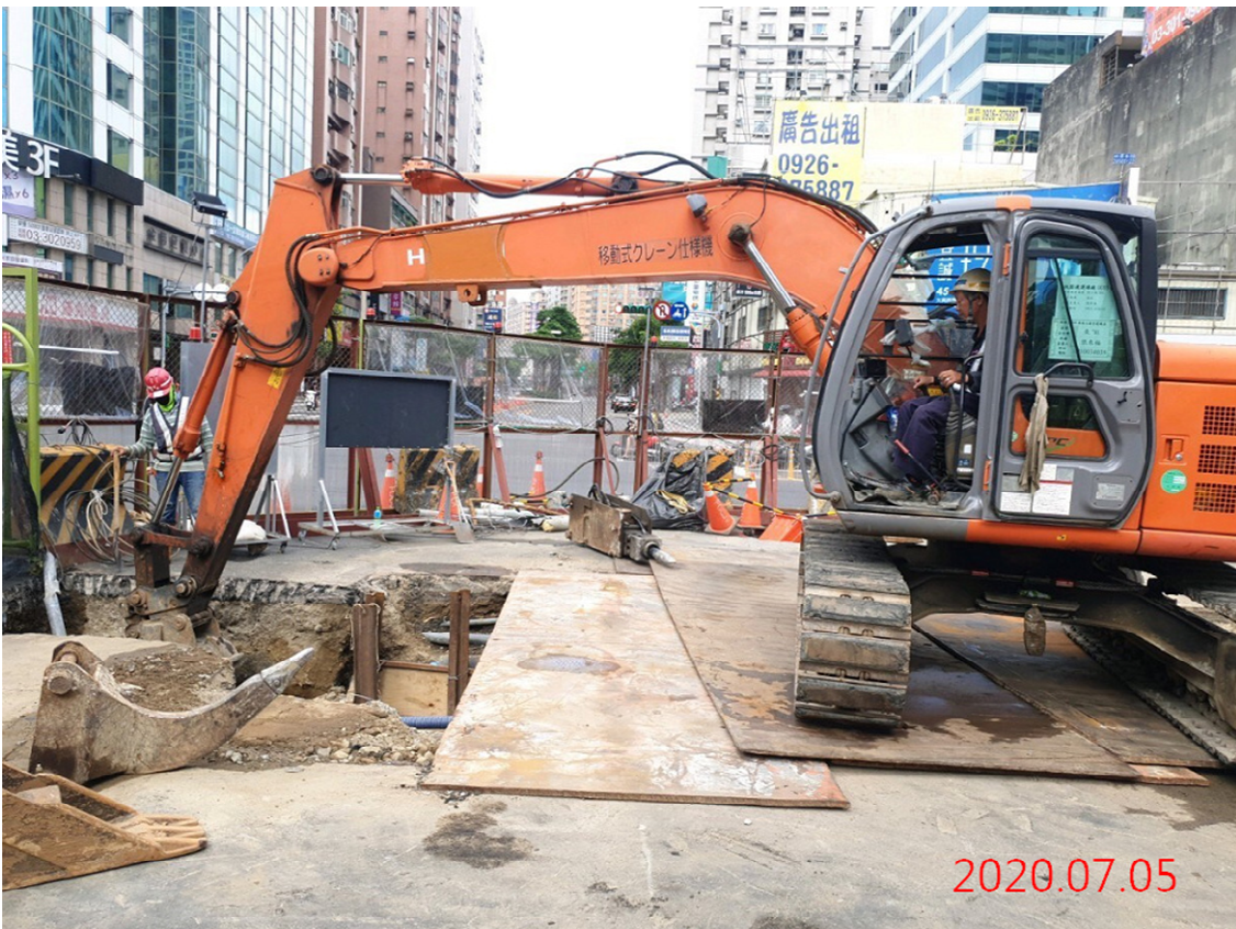
G10 站_管線探挖
