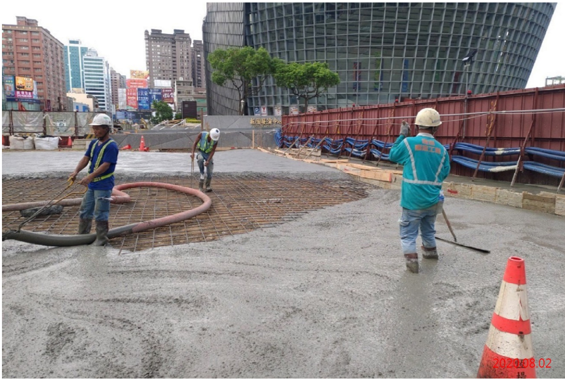
G11 站_南工區鋪面澆置
