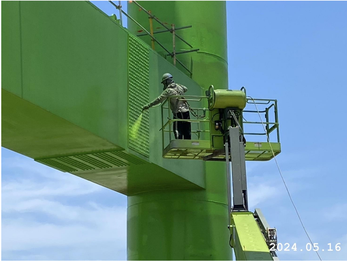
DU14-14 鋼箱樑補漆
