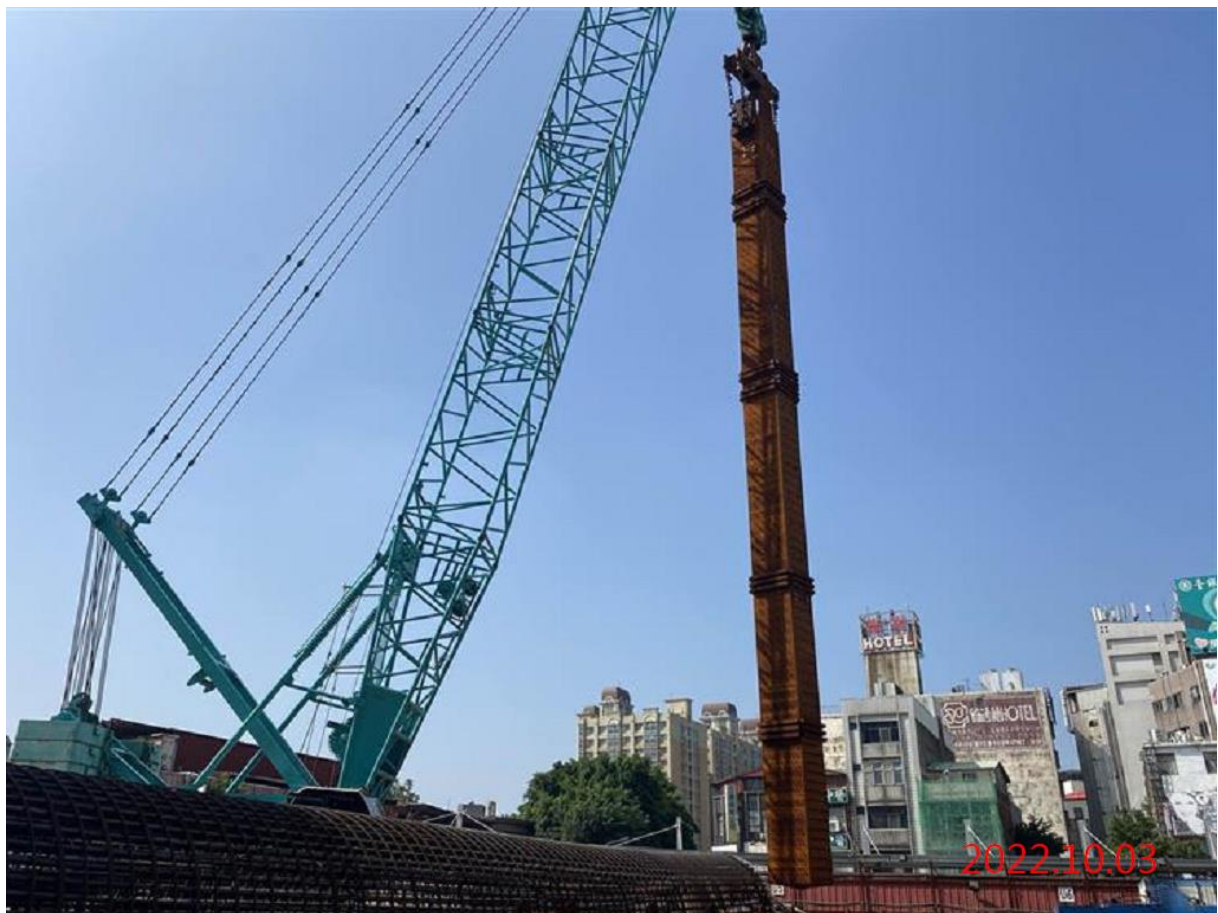
G07 站_全套管基樁逆打鋼柱吊放
