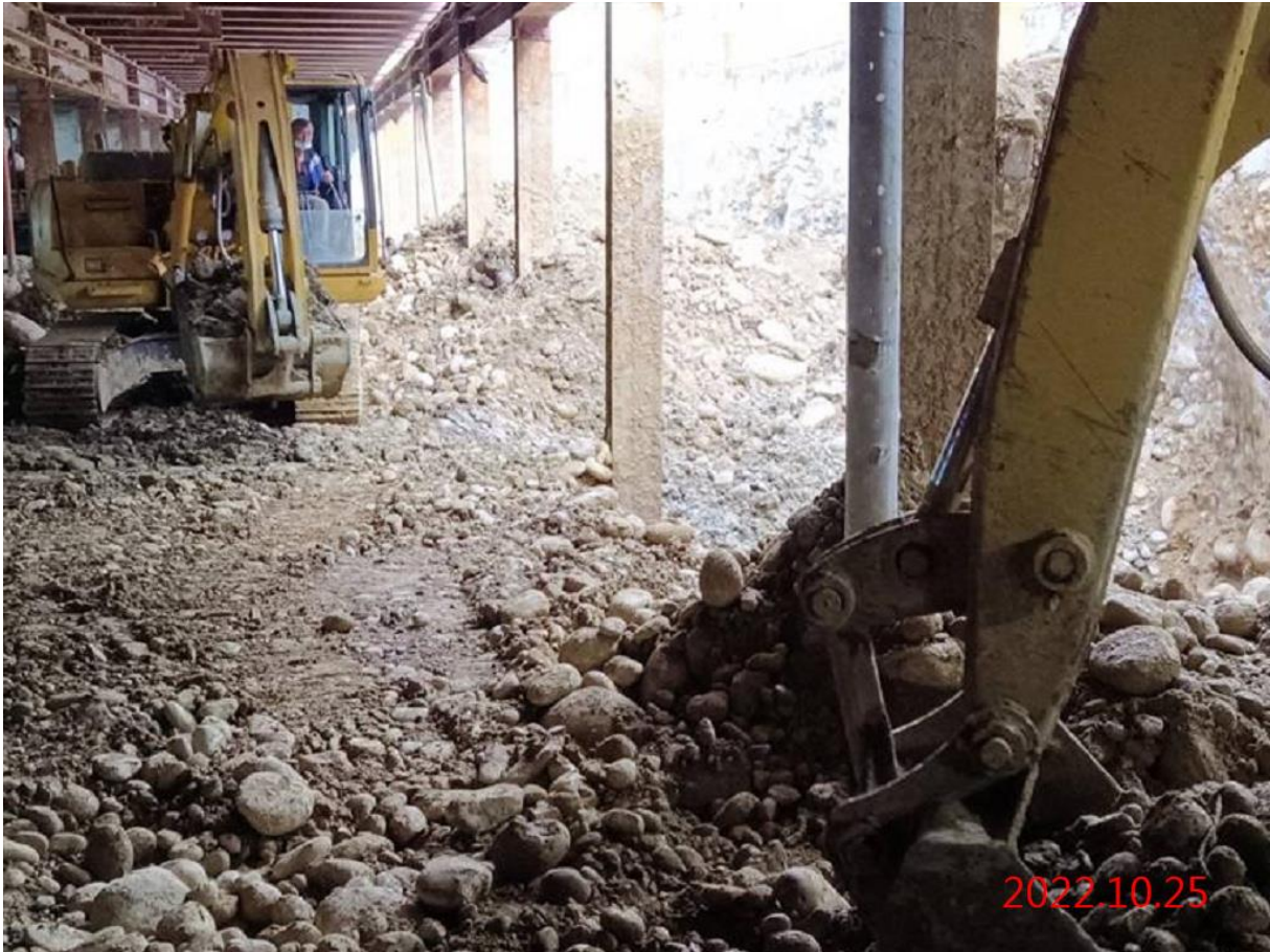
G11 站_站體出入口開挖
