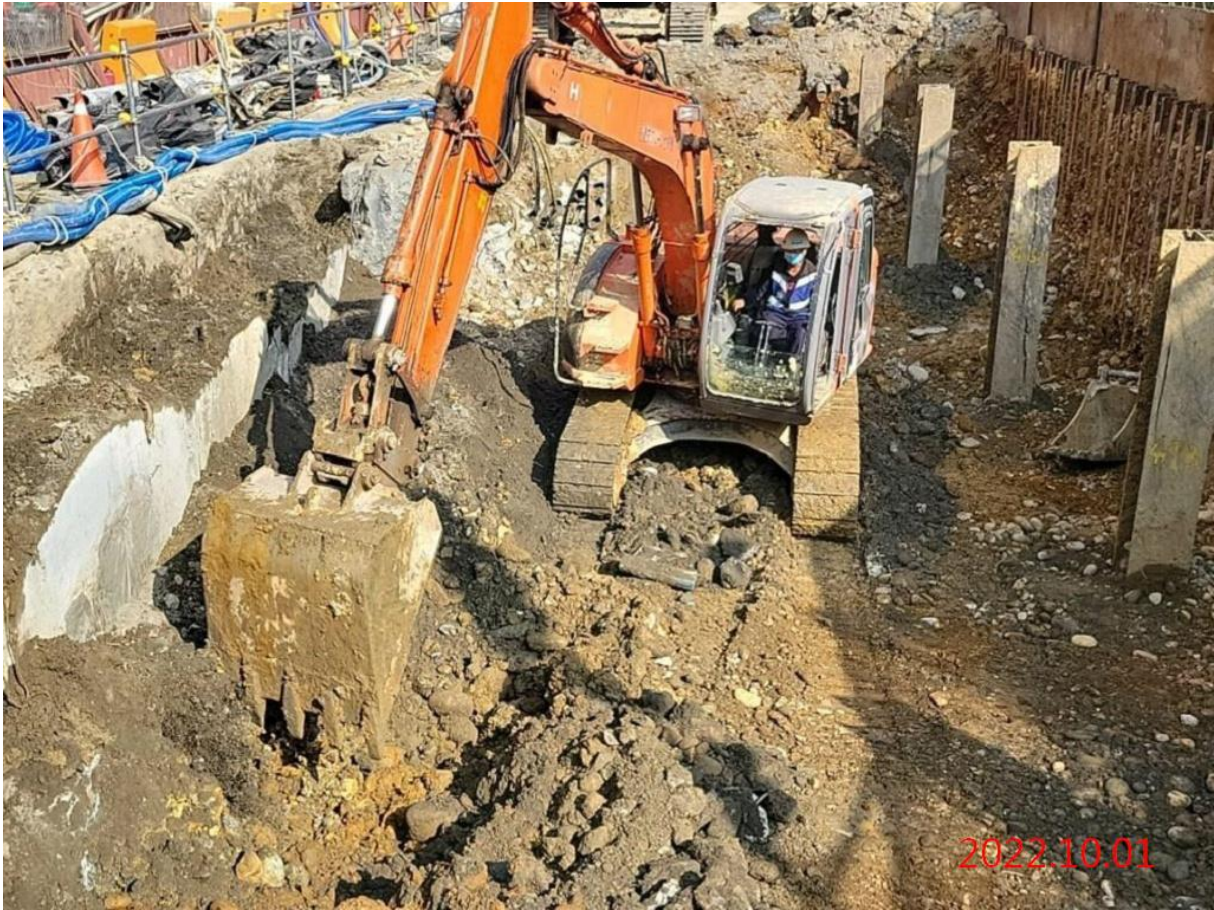
G10 站_站體開挖
